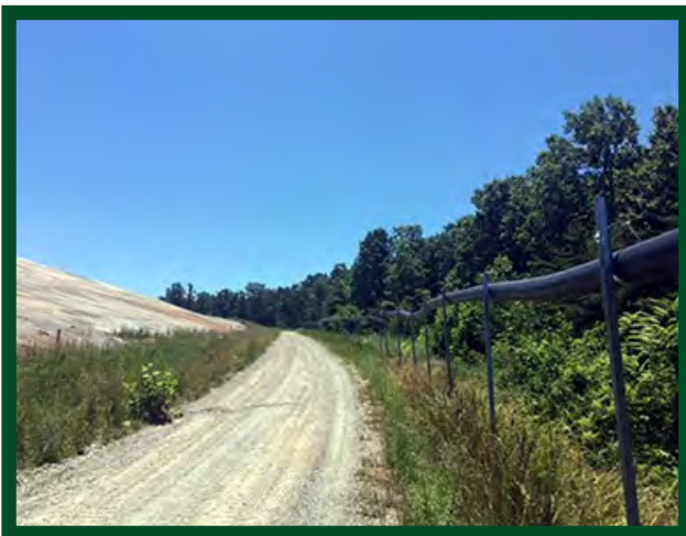
Vapor-Phase Perimeter Odor Mitigation System Surrounding the Perimeter
