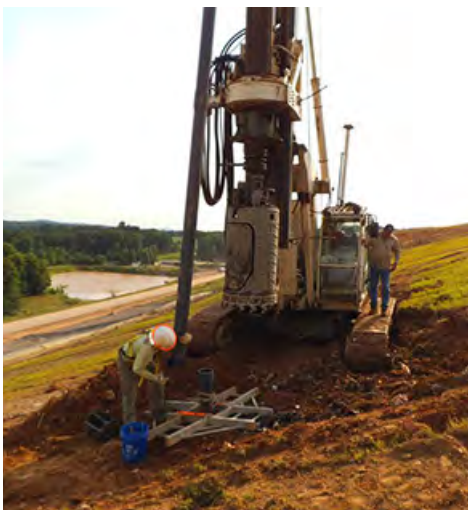
Landfill gas extraction well
