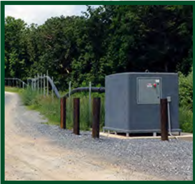
Vapor-Phase Perimeter Odor Mitigation System
