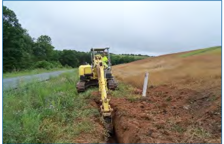
Installation of pilot gas collection system at the Livestock Road Regional Landfill.
