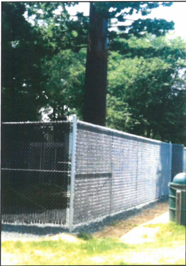
Fenced in equipment before landscaping.
