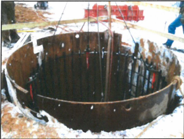
First the foundation of the tower is drilled. A metal casing is used to pour the concrete base.
