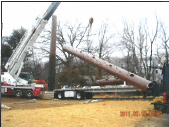
The second part of the pole is lifted with a crane and carefully attached to the “trunk.”
