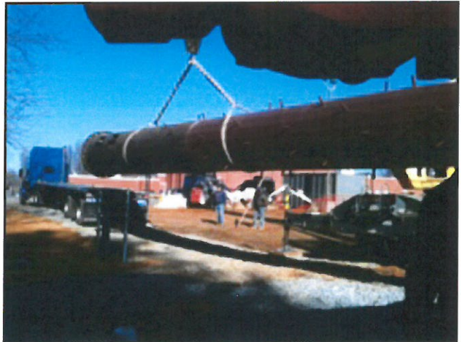
The first part of the pole is then attached to the steel and anchor bolts are embedded in the concrete foundation.
